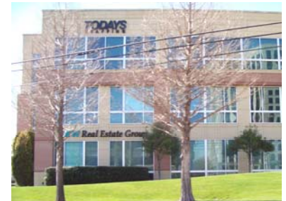
Preston Rd. Office Corridor
