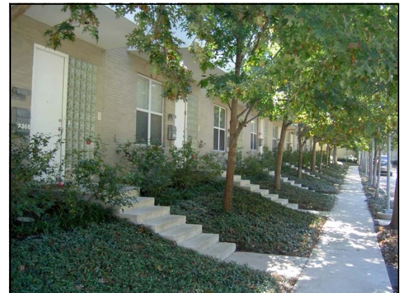
Figure 1. EXAMPLE OF INCAP REDEVELOPMENT PROJECT
