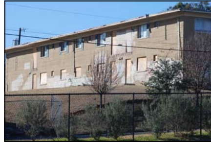
Figure 2. CHATEAU CREEK APARTMENT BEFORE DEMOLITION
