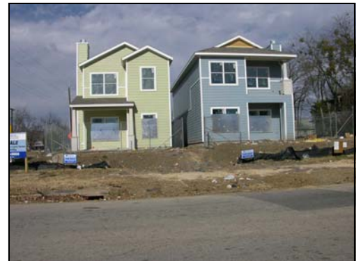
Figure 1. NEW HOMES UNDER CONSTRUCTION NEAR FAIR PARK
